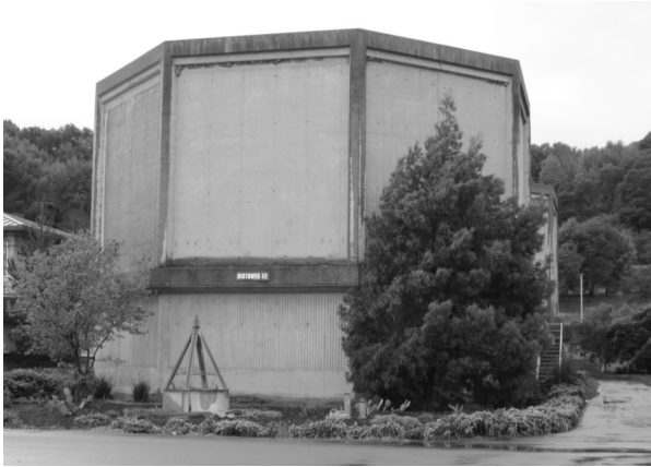
The untreated waste water filling this bio tower at Central Marin Sanitation Agency will be converted into water that can be released into the bay through an organic treatment in which bacteria in the plant eat the waste, or nutrients, in the raw sewage.
